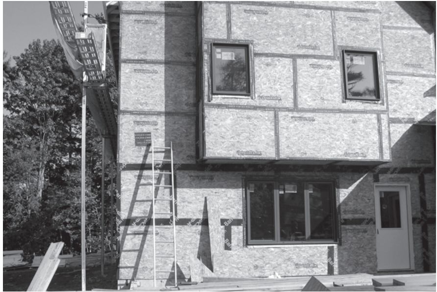
Example of exterior-sheathing air barrier strategy, with primed and taped sheathing joints. Coldham & Hartman’s project for new dorms, College of the Atlantic.
