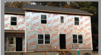
Insulated sheathing with taped seams is an excellent primary air barrier.
