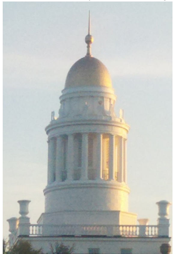
Pittsfield High School Dome Restoration
