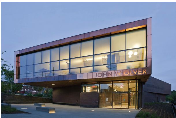
JOHN W. OLVER TRANSIT CENTER: June 2015 Greenfield MA, the first Zero Net Energy transit center in the country – Charles Rose Architects
