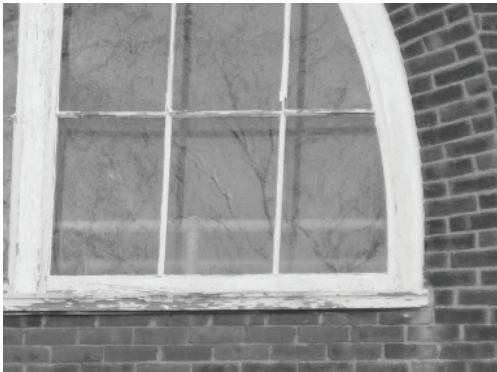
CLOSE UP OF DAMAGE TO HISTORIC WINDOW
