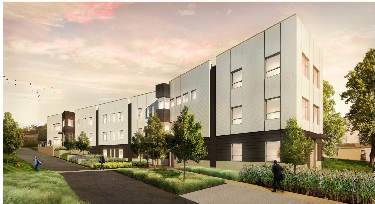
Crotty Hall is a 16,500 sf building currently under construction at 418 North Pleasant Street in Amherst. It is designed to be a net-zero energy facility that will house faculty and graduate students in the Department of Economics at UMass Amherst. It is sited with the intention of creating an "economics campus" in conjunction with Gordon Hall which already accommodates a portion of the faculty in economics.
