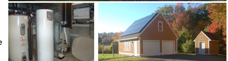
2004 Solar HW tank, new Stiebel Eltron heat pump hot water heater, Daikin air source heat pump furnace unit, and Renewaire ERV.
