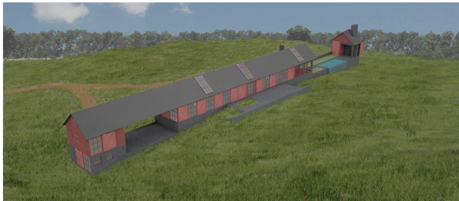
We took the familiar barn form and stretched it to new lengths. Our clients wanted to leave the field as untouched as possible, so all landscape is contained within the 24' width. The roof is continuous over the 300 foot span, with one gap for the pool and associated recreational spaces. The parking and garage are under the covered roof. The two small buildings at the two ends house the guest house and the pool house.
