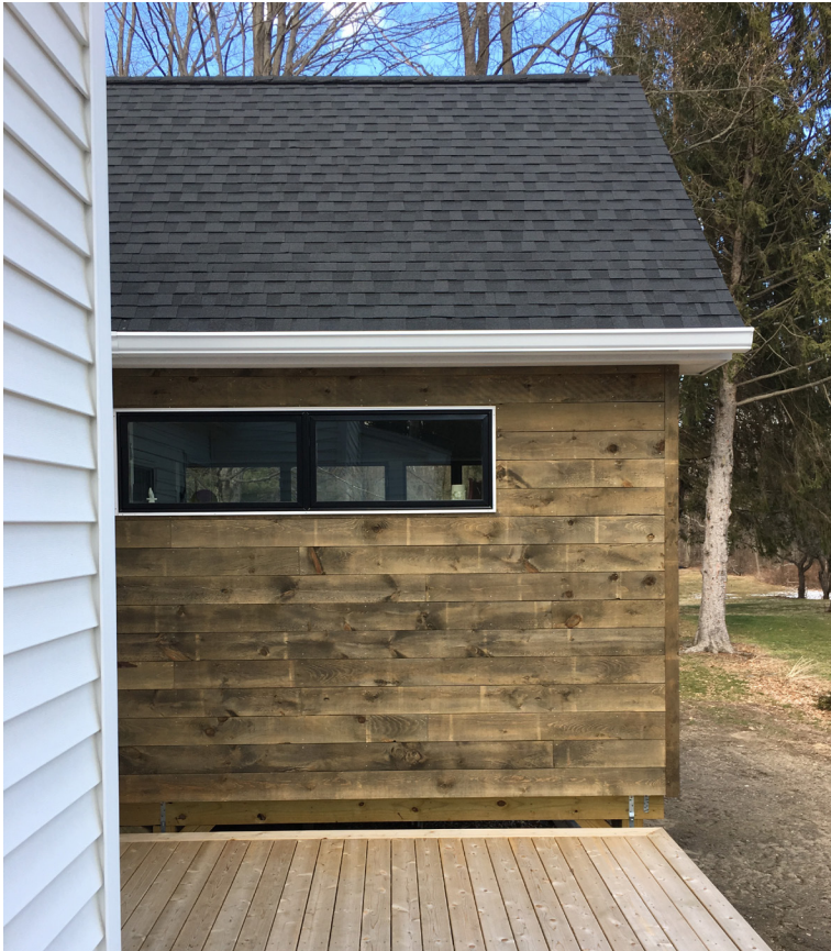
Rough sawn, ship-lapped pine from Vermont with a transparent stain finish is the exterior cladding at the new addition. A double 2x4 framed wall with dense pack cellulose insulation and a 1" vented air space make up the rest of the exterior wall system.
