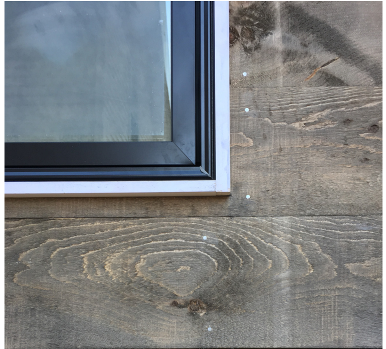
Rough sawn, ship-lapped pine from Vermont with a transparent stain finish is the exterior cladding at the new addition. A double 2x4 framed wall with dense pack cellulose insulation and a 1" vented air space make up the rest of the exterior wall system.
