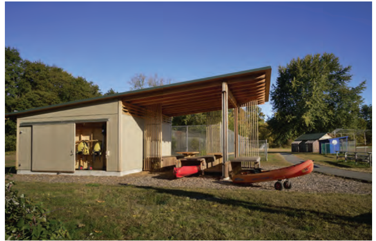
R: South side of Kiosk showing storage for the life jackets and paddles. Restroom is beyond the blue dugout.
